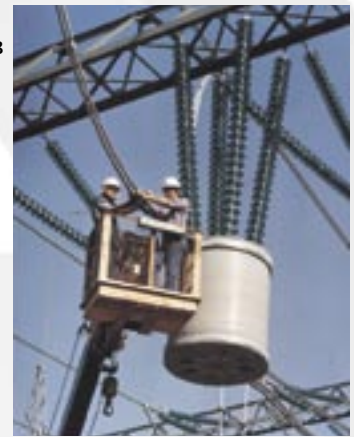
500kV suspension mounted line trap
