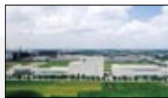
Trench® China - Shanghai
